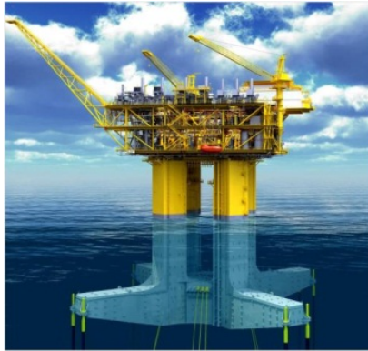
Figure 4: Tension leg platform
