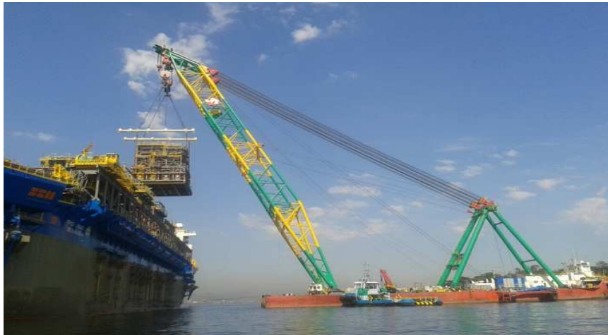
Module lifting FPSO Ilhabela – 2014
