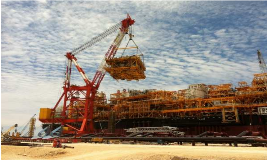
FPSO CLOV (Total) module lifting – 2013
