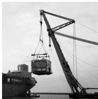
Top: Process facilities on FPSO Capixaba Bottom left: Semi-submersible production platform Thunder Hawk on location Bottom middle: Typical process module fabrication Bottom right: Lift of a module onto FPSO P-57 for Petrobras
