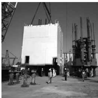
Top left: Semi-submersible production platform Middle left: Offshore workers replacing a gasket Bottom left: Wind turbine installation vessel during commissioning of jack-up system Top right: Lifting operation of crane house of the 5,000 tonnes of crane Bottom right: Construction workers in Singapore
