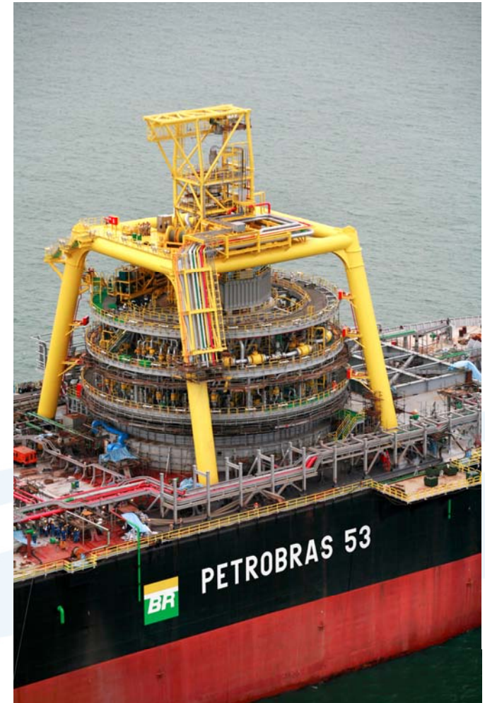
'P53' internal turret completed
