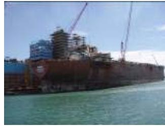
Woodside - FPSO Okha
