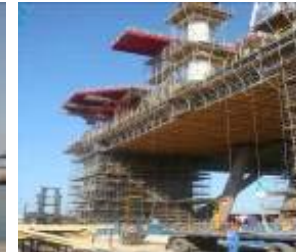
Odebrecht - Drilling Rig
