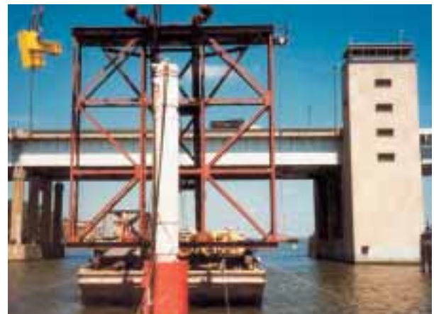
The S-500 Hydrohammer, used at the Woodrow Wilson Bridge, USA.
