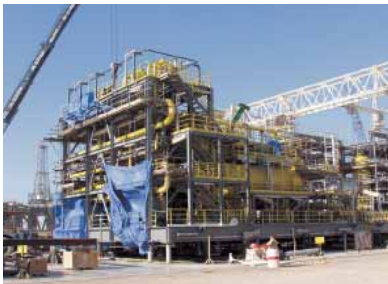
Two of the main modules for Xikomba FPSO, under construction.
