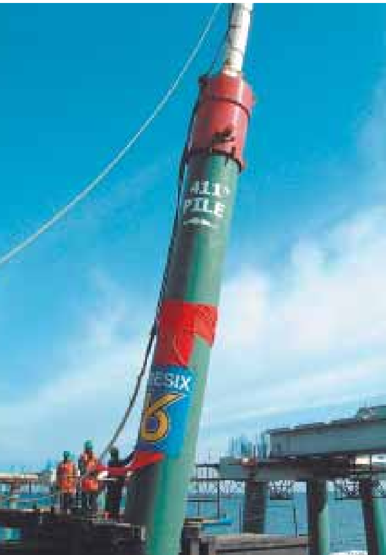
IHC Hydrohammer – Last pile at the Wafa coastal plant, Libya
