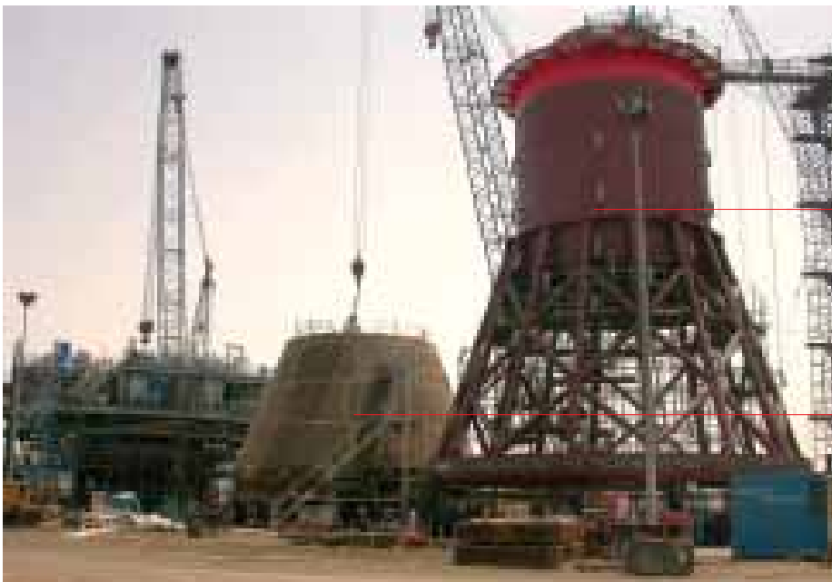
White Rose turret components being constructed in GPC Dubai
