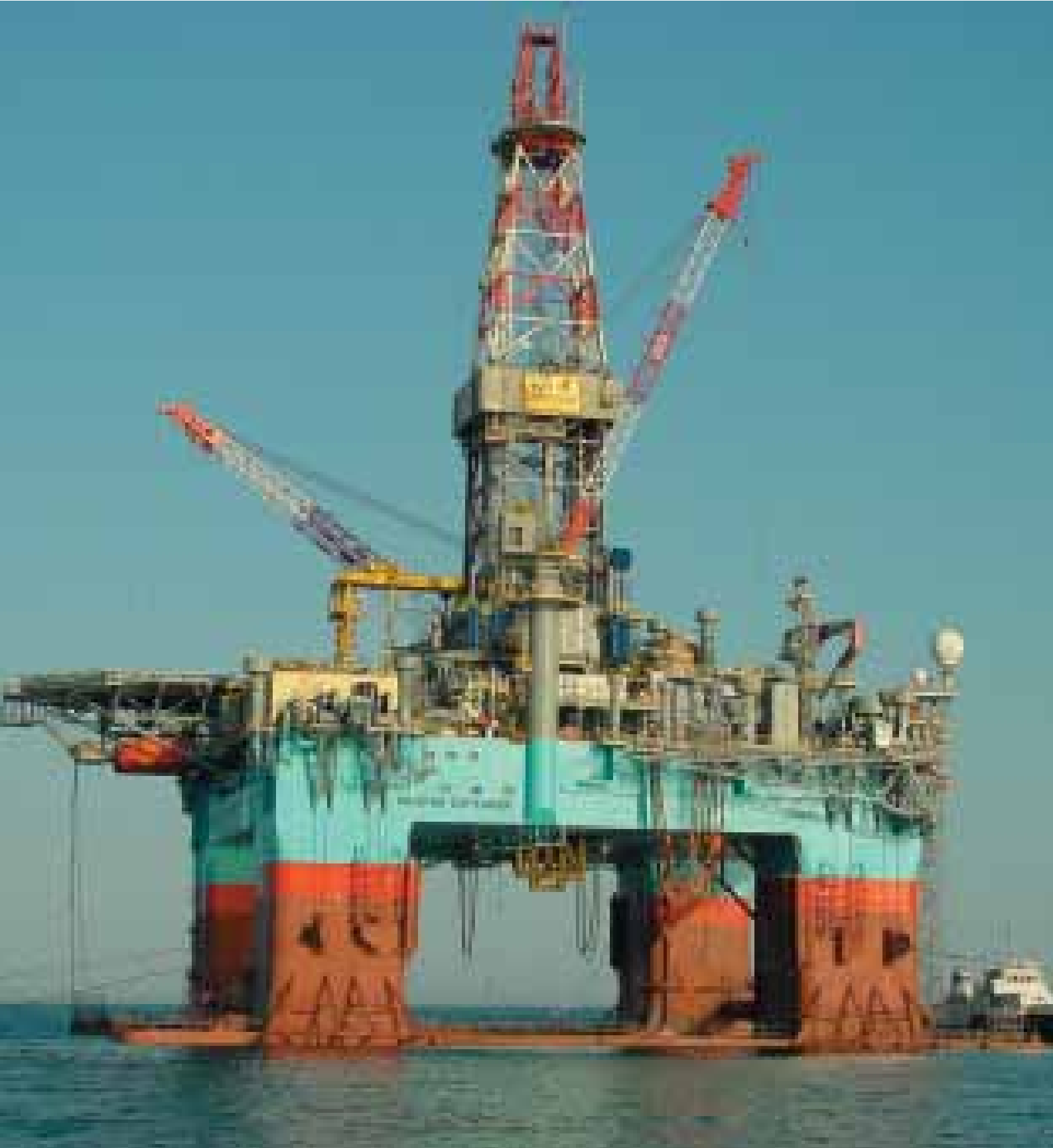
MSC – Maersk Explorer during commissioning in the Caspian Sea
