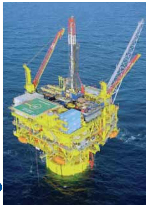
Dry-tree SeaStar® TLP in production on Total's Matterhorn field, Gulf of Mexico
