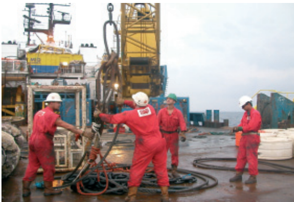
Work on deck of the 'Dynamic Installer' during a CALM buoy installation
