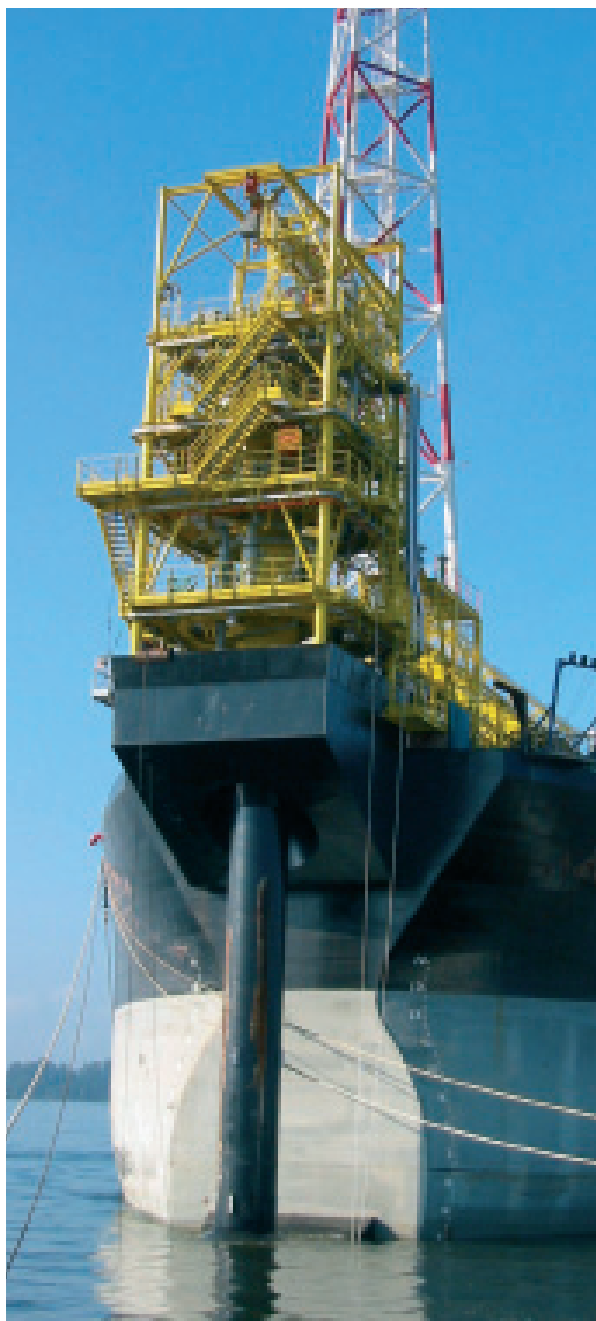
The external turret mooring system of the 'Bunga Kertas' FPSO of MISC
