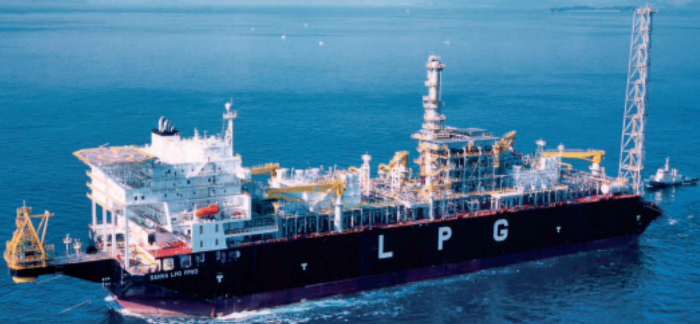
The Sanha LPG FPSO on departure from the construction yard in Japan en route for Angola
