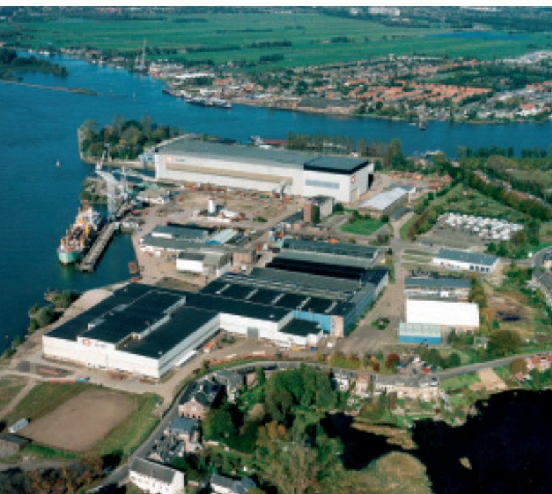
The yard of IHC Holland in Kinderdijk
