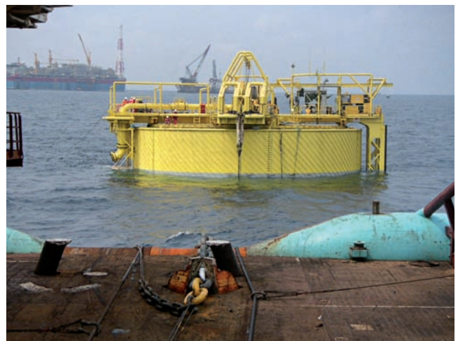
A scale model of the deepwater export CALM for the Erha field of ExxonMobil and the installation of the buoy offshore Nigeria
