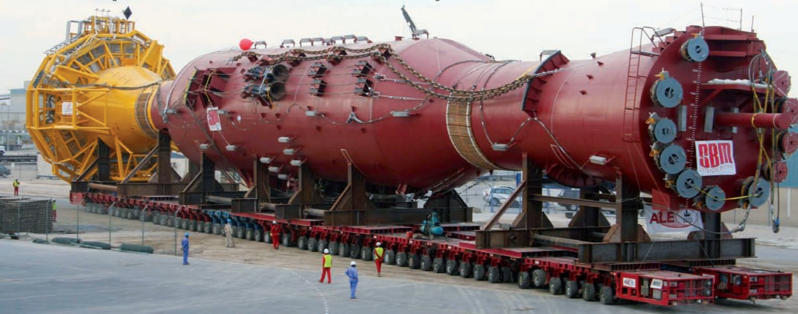
The mooring column of the external disconnectable turret for the Enfield FPSO during load-out
