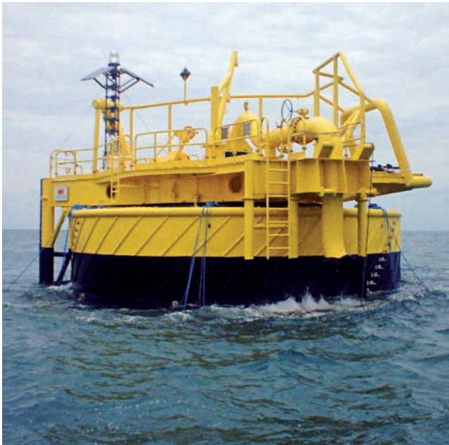
CALM buoy for Trafigura installed at the Tema refinery in Ghana
