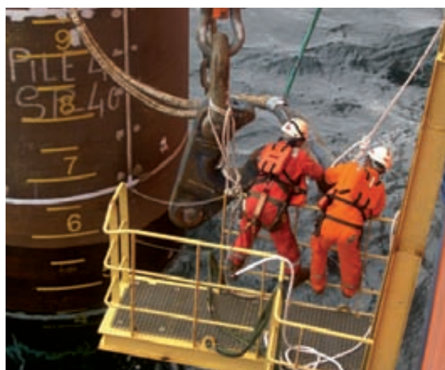
Installation of the Anchor piles for FPSO Mondo, offshore Angola
