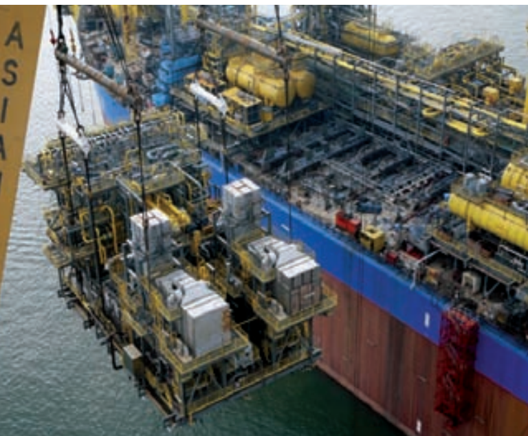
Module lift onto the deck of the FPSO Saxi Batuque
