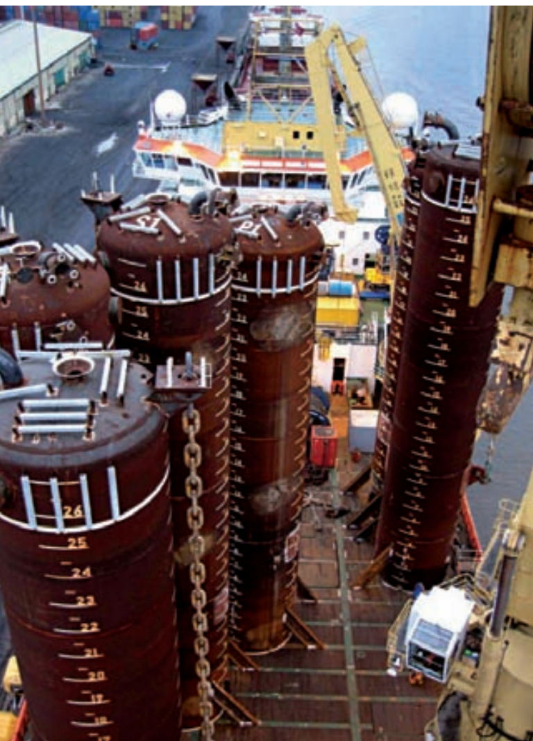
Suction piles for Agbami FPSO on 'Normand Installer' for installation
