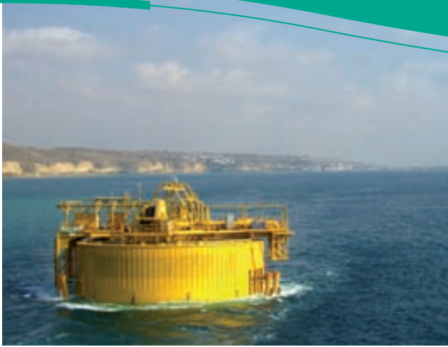
Tow of the deep water CALM buoy for Greater Plutonio FPSO for installation offshore Angola
