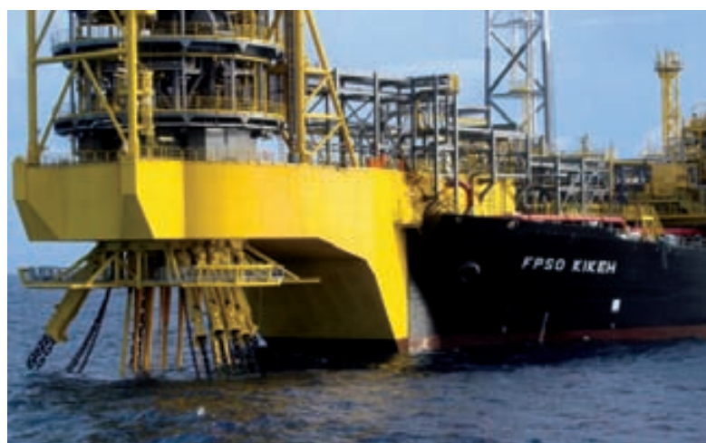
FPSO Kikeh external turret
