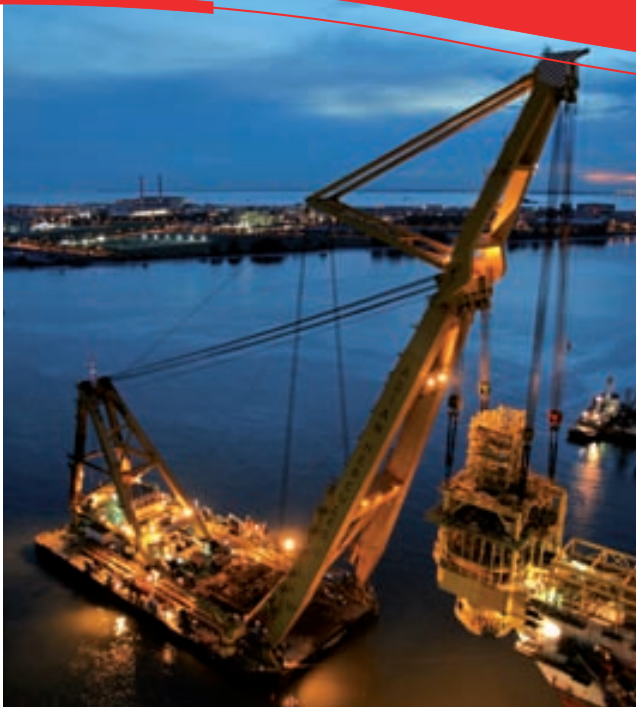
Heavy lift of the external turret for FPSO Saxon Batuque
