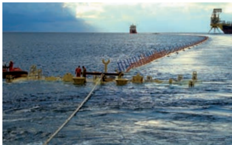
GAP™ during installation on the Kikeh Field, Malaysia
