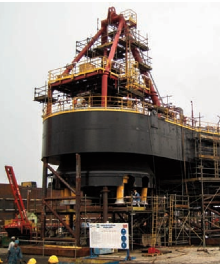
Su Tu Vang external turret during construction
