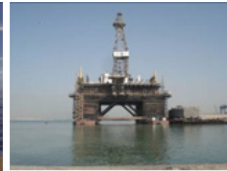
QGP - Drilling Rig
