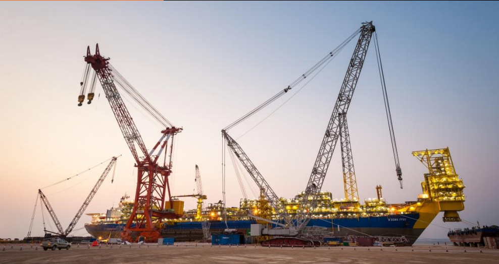
FPSO N'Goma (12 year L&O contract)
