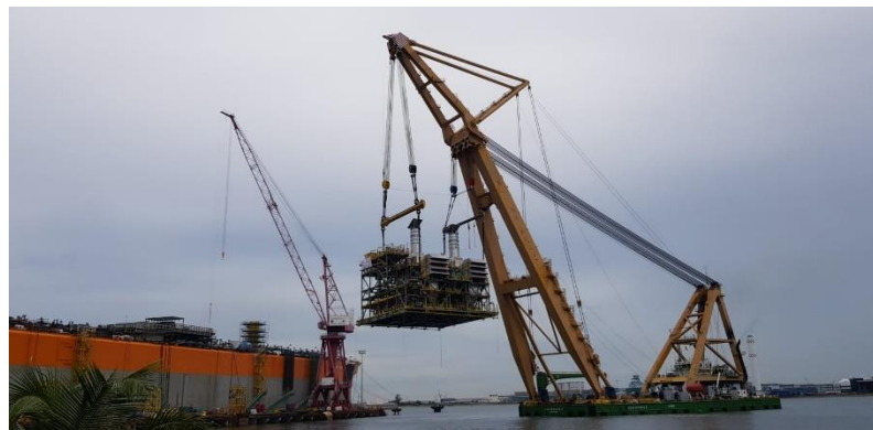
Module lifts Q4 2018
