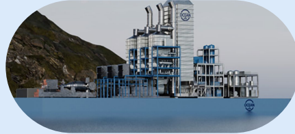
Floating Power Hub
